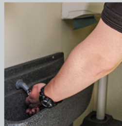
Delivery of hot water
