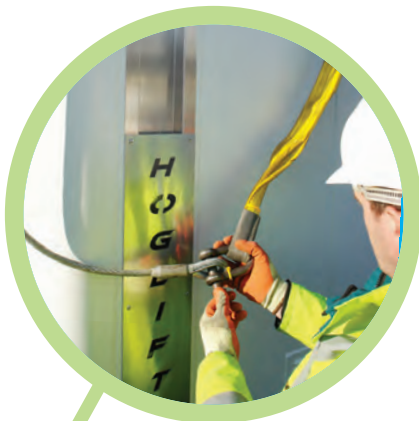
4 Attach slings to rear lifting hook, and repeat process for the front
