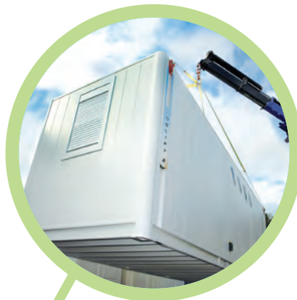
5 Elevate unit and position at ground level
