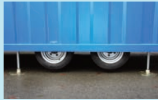
Rams lift unit from ground ready to release axle pins
